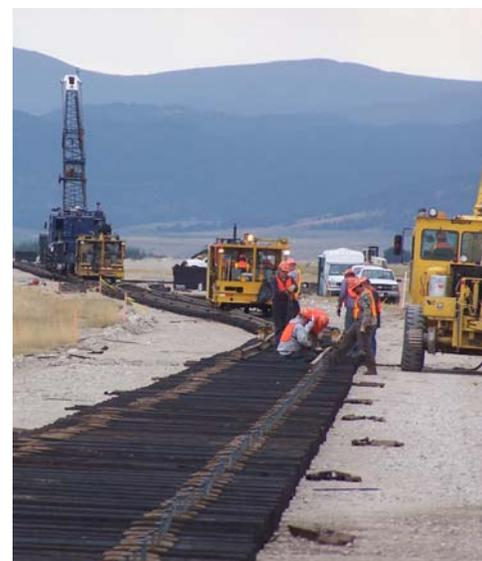
Montana Rail Link workers installing track to the BP/ARCO repository at the Anaconda Smelter Superfund Site.
