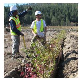
Work Crew (above) installing logs pre-planted with willow and alder species. Several rows will be placed perpendicular to the stream channel to provide floodplain stability. Also visible are stumps from the dam construction (1905-1908).
