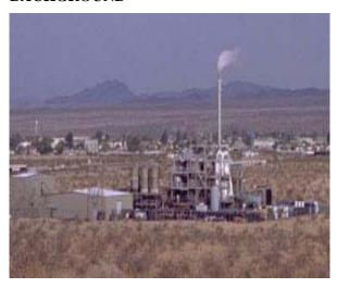
Westates is a hazardous waste storage and treatment facility located near Parker, Arizona on the Colorado River Indian Reservation. Westates treats spent carbon in a furnace to remove contaminants from the carbon. The contaminants are then processed through various Air Pollution Control Devices (APCDs) prior to being released to the atmosphere.
