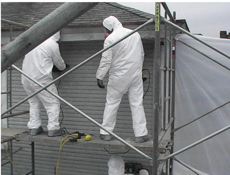
**Figure A-7. Power grinding paint from 2<sup>nd</sup> story wall**
