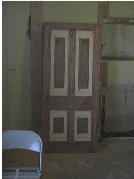
**Figure A-2. Door with paint removed**
