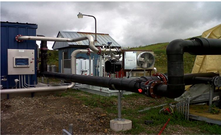
The facility currently uses approximately 350 standard cubic feet per minute of landfill gas with an average methane content of approximately 52%. The methane gas is chilled prior to sending it in the transmission pipeline to the CARES facility using a multistage centrifugal blower. The landfill gas is regulated into either of two 9.8 million BTU low pressure steam boilers at roughly 2 psi. The boiler manifolds were modified to support beneficial use of the landfill gas.
