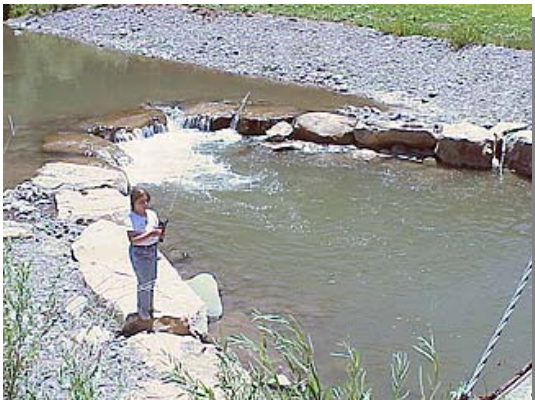
Aquatic habitat was improved by adding a drop structure. The pool in this area is 7 feet deep and supports trout.
