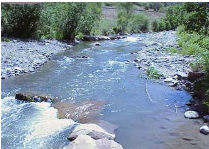
The J-hook in the foreground is typical of the structures installed in the river. It directs stream flow toward the thalweg and away from the banks.
