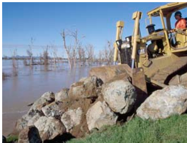
A flood-damaged levee on the Feather River was repaired in 1998
