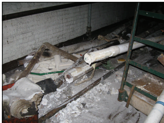
The pipe room where employees were directed to store pipes containing asbestos contaminated materials after illegally taking them down.
