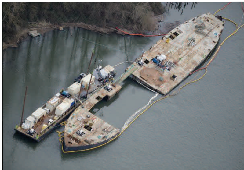
The Davy Crockett, shown in an aerial view last March, was surrounded by a cofferdam and dismantled in place.
