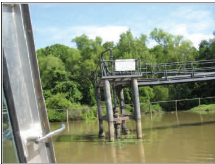
The underground injection well operated by FAS. This is a Class II well, permitted by Louisiana Department of Natural Resources.
