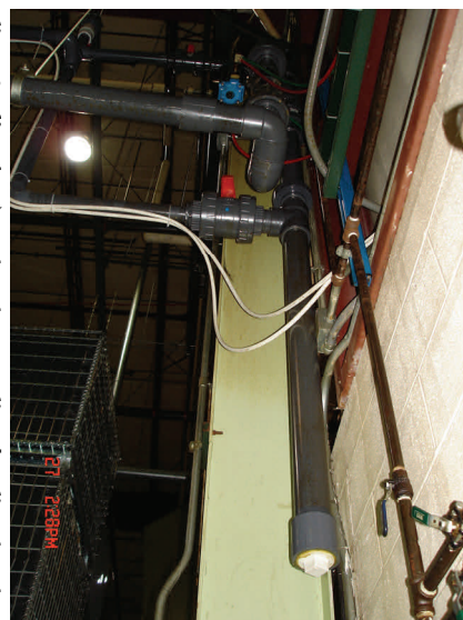
Cut illicit discharge pipe
