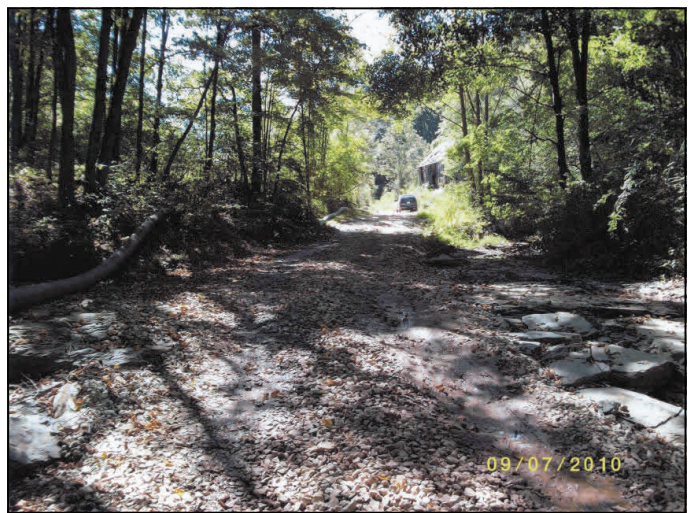
Blake Fork after having stone and gravel spread in the stream to create a roadway
