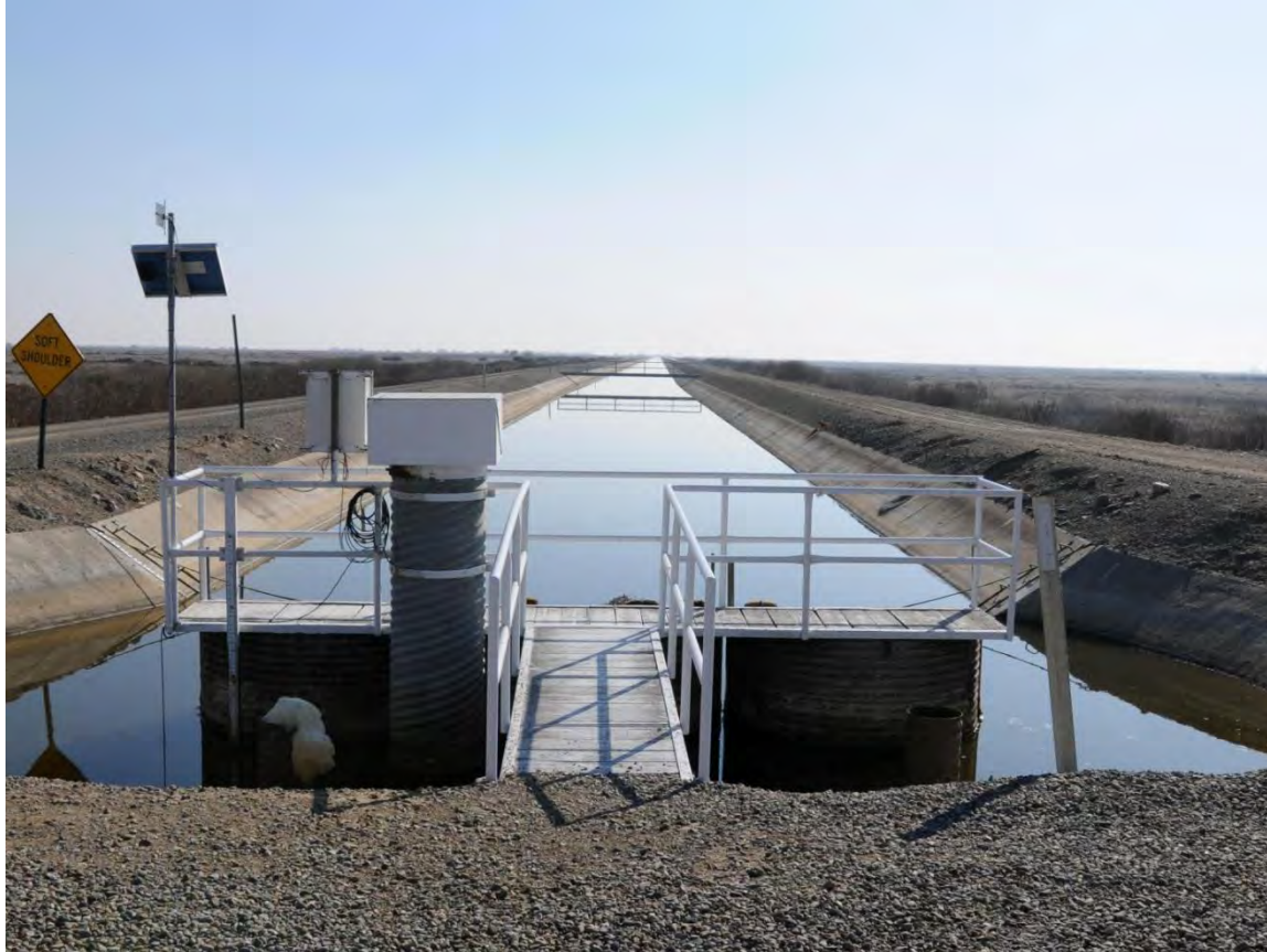
GBP Selenium Drainage in San Luis Drain Before Discharge to Mud Slough
