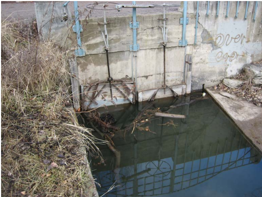
Orchard Homes irrigation ditch head gates.
