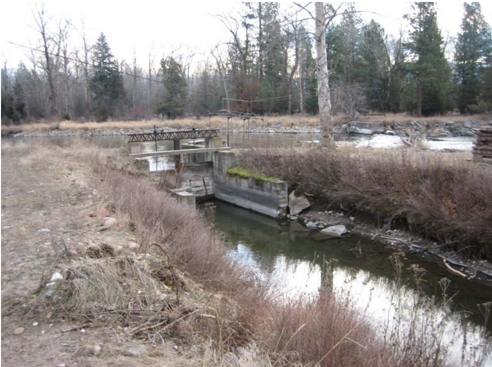
Head gates to the Grass Valley irrigation ditch from channel.
