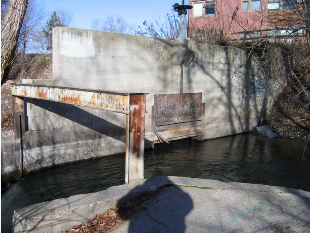
Head gates of the Flynn-Lowney irrigation ditch.
