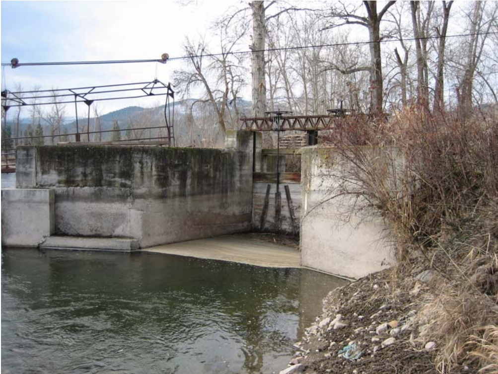
Head gates to the Grass Valley irrigation ditch from CFR.
