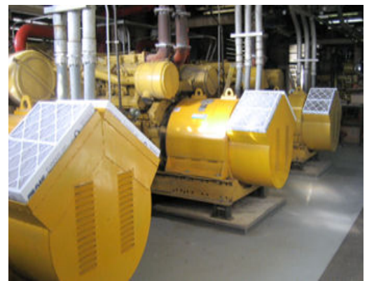
Figure 9. An example cogeneration system that resembles the one found at the City of Santa Cruz Waste Water Treatment Plant.
