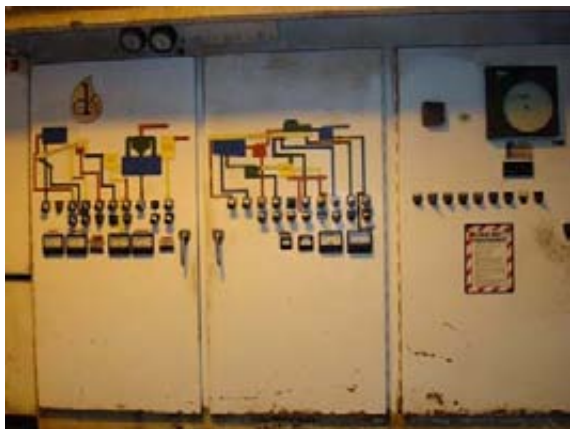
Control Panel for Pretreatment Processes
