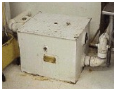
Figure 2. Picture of an interior grease trap. Small grease traps are sufficient for low volume producers and may require as frequent as weekly maintenance.
