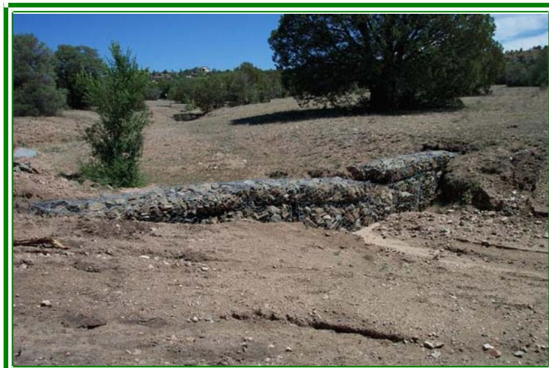
Yavapai-Prescott Indian Tribe protecting water quality by preventing erosion with a gabion structure in an eroded drainage area.
