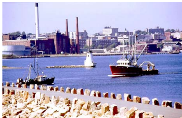
New Bedford shoreline with hurricane barrier in foreground. Photo by C. Pesch
