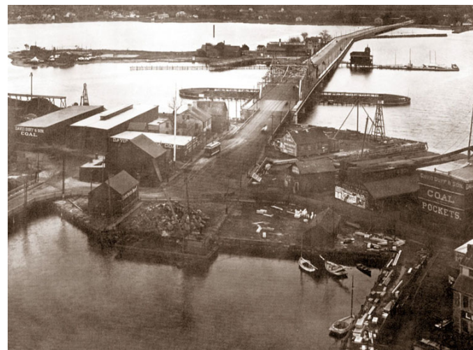
The original bridge was destroyed by the Gale of 1869 and rebuilt in 1870. The wooden bridge was replaced by steel in 1898. This photo by Joseph G. Tirrell, taken c. 1900, shows the bridge under construction. The view is east toward Fairhaven, with Fish Island in the foreground. The western section of the bridge, from New Bedford to Fish Island, had not yet been completed. Courtesy of the New Bedford Whaling Museum.
