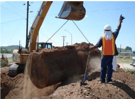
An Underground Storage Tank being lifted from the ground
