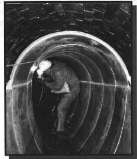
Sewer rehabilitation can include lining aging sewers (photo: NJ Department of Environmental Protection).
