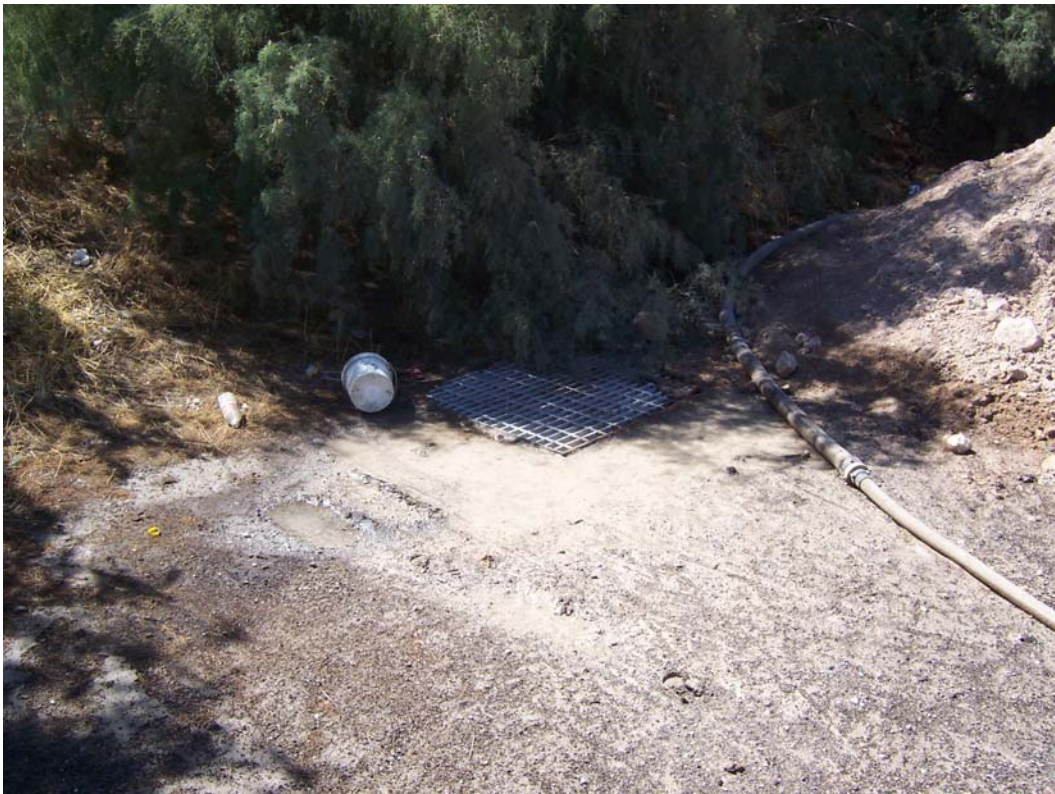
Photo 5. Storm inlet located behind the pile of dirt shown in Photos 3 and 4. Note contaminated runoff from the site entering the inlet.
