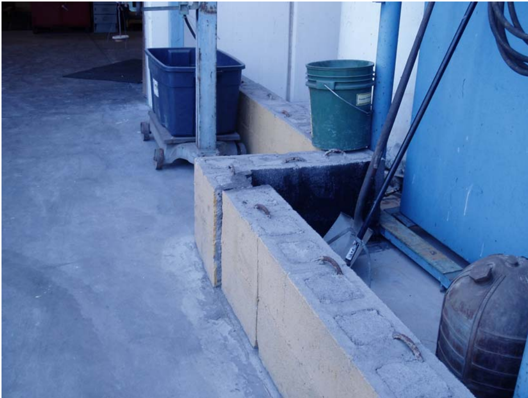
Photo 1. Crack in secondary containment.
