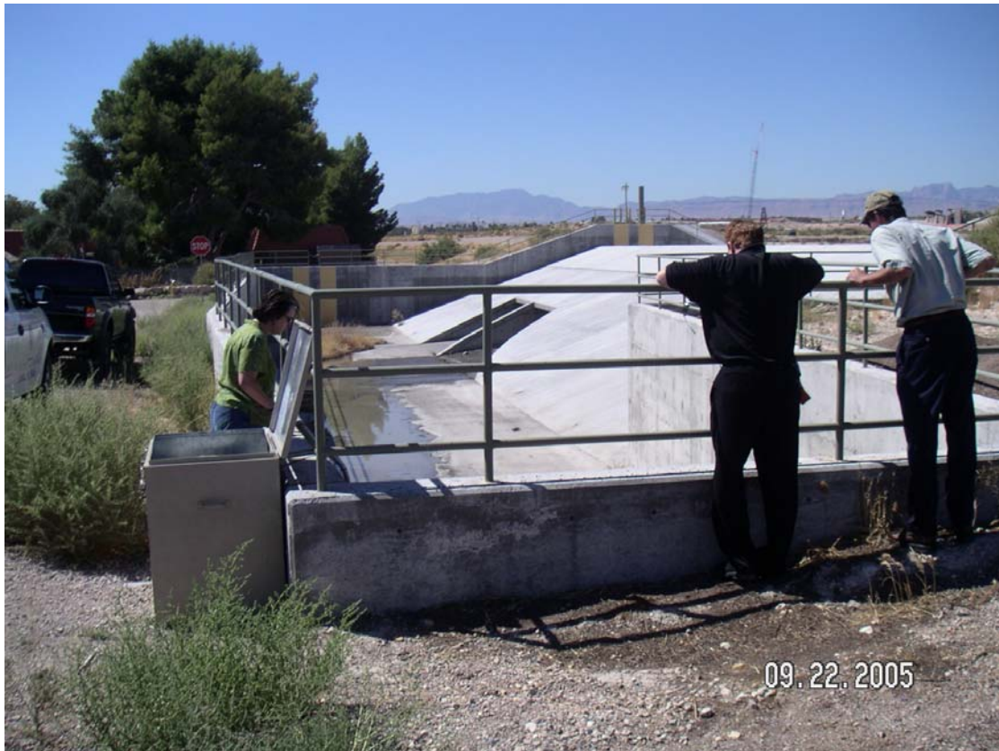
Photo 13. Meadows Detention Basin - effluent sampler and outfall.
