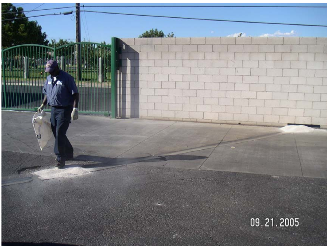
Photo 4. Worker spreading absorbent material.
