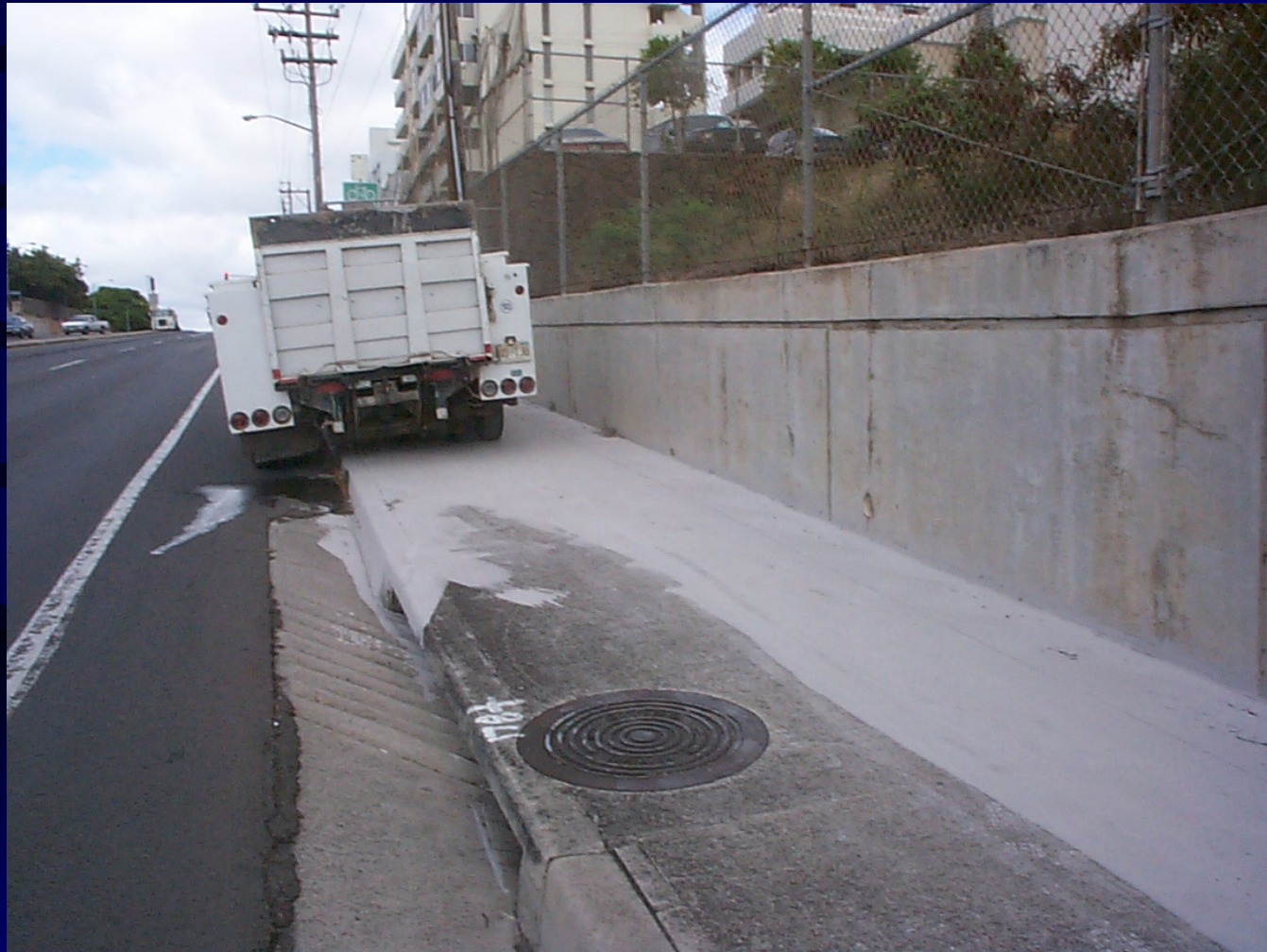
Storm Drain Protection
