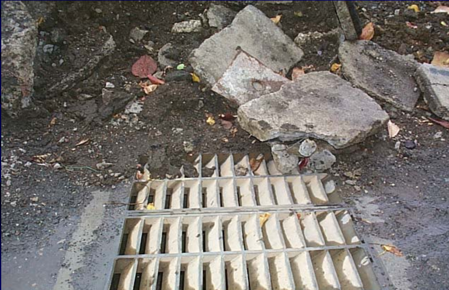
Storm Drain Protection
