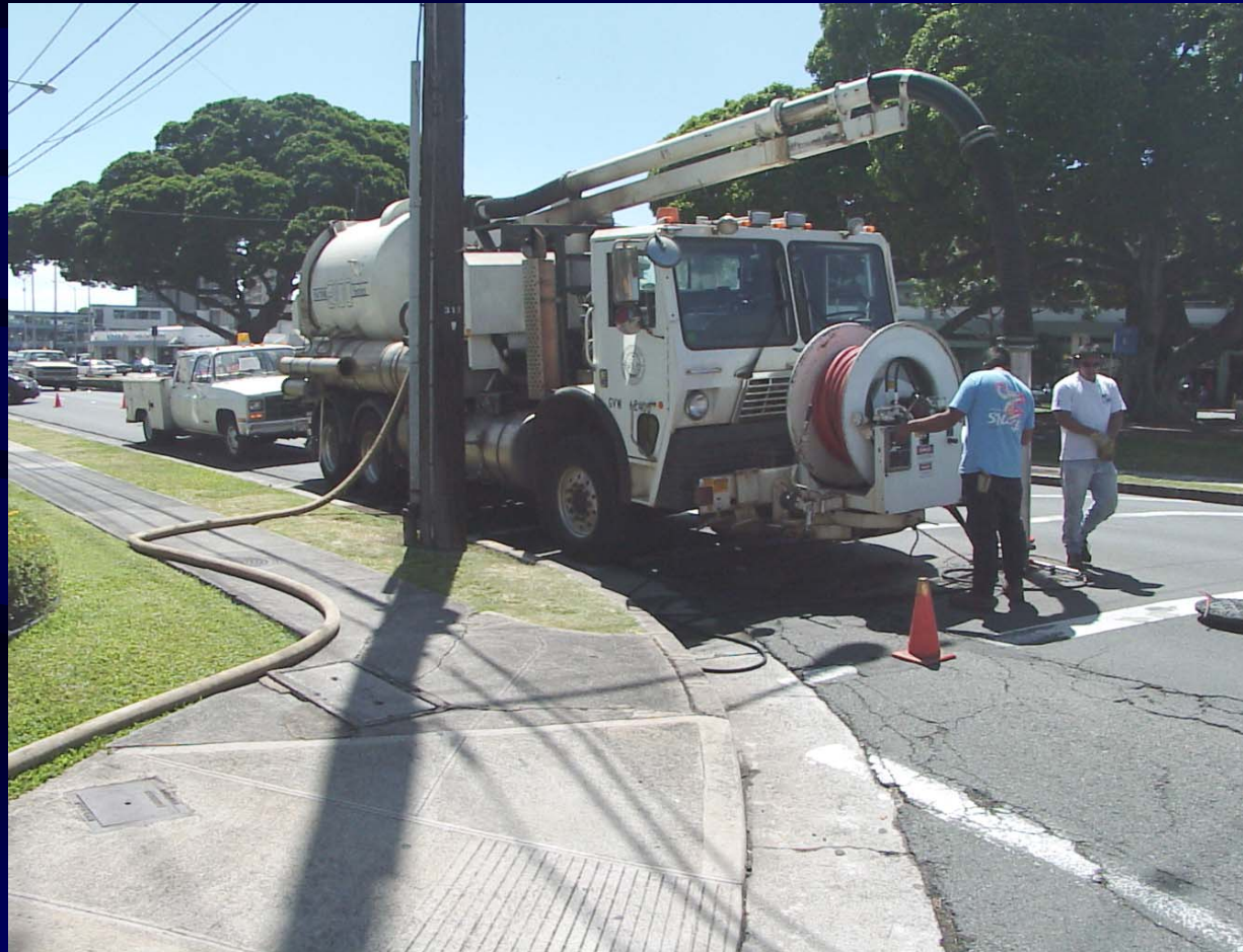
Storm drain maintenance with vactor trucks
