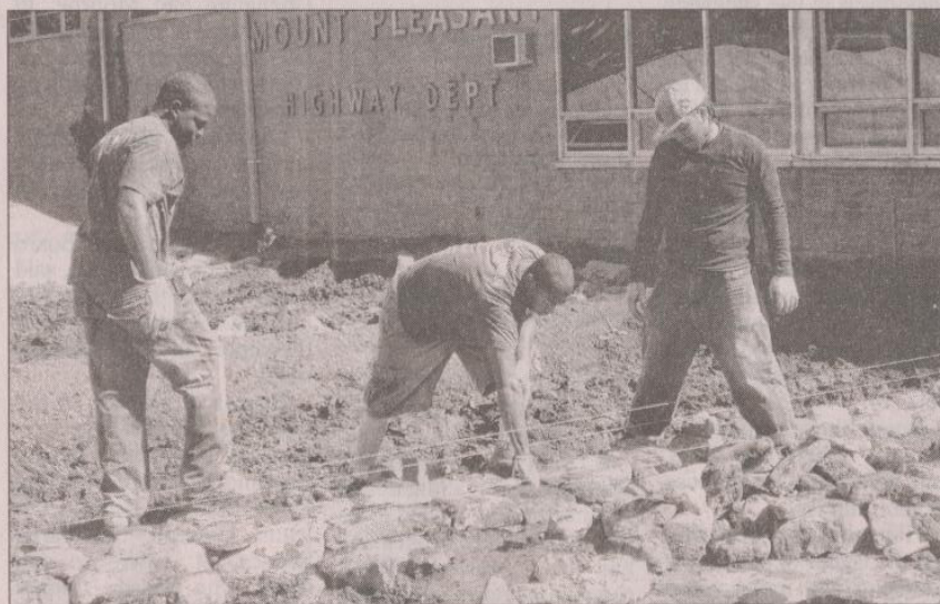
A team of stone wall builders from Groundwork Hudson Valley set up the borders for a rain garden outside the Mount Pleasant Highway Department on Wednesday. The organization is using federal and state grant money to provide the town with natural stormwater control to cut down on flooding and pollution in the nearby Saw Mill River.
