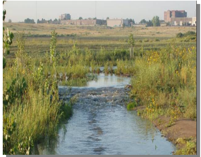
Grade-control structures designed to emulate natural stream riffles using a mix of rock observed in a tributary to Cottonwood Creek.
