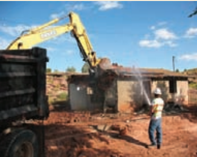
Demolition of contaminated home
