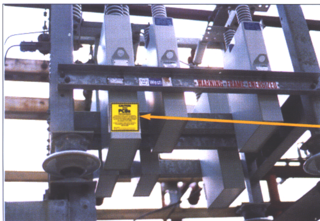
Looking up at PCB Marked Capacitor on the left (graphic below)
