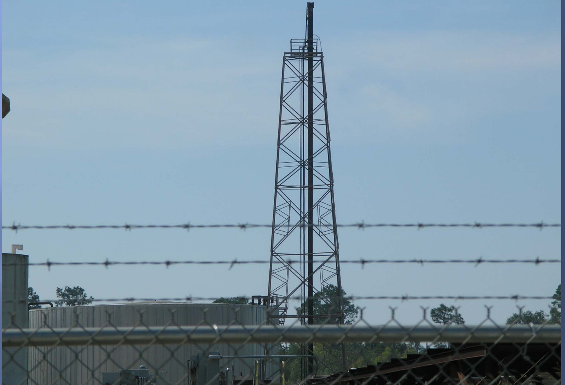
Exhibit 14. Process Flare Stack.
