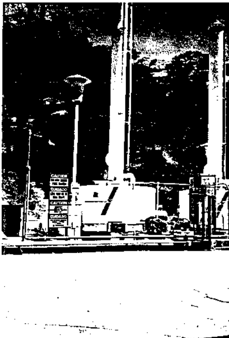
1-O. Air Stripping Towers for Groundwater Treatment at Bowl Area. (SWMU 4.18)
