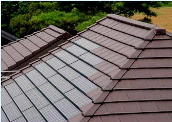
Building integrated PV. Image courtesy Kyocera 22
