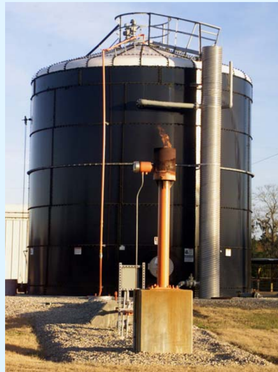
Fixed-film digester. Image courtesy University of Florida 52
