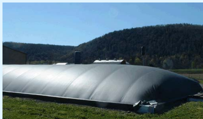
Plug flow digester. Image courtesy Penn State University 53
