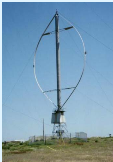
Darrieus model wind turbine. Image courtesy Solcomhouse 29
