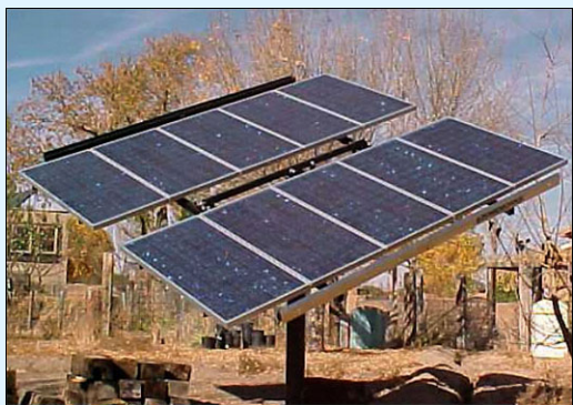
Solar Tracking Unit. Image courtesy Northern Arizona Wind and Sun 17
