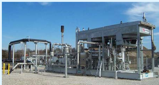
Landfill gas treatment/blower/flare station. Image courtesy LMOP 40
