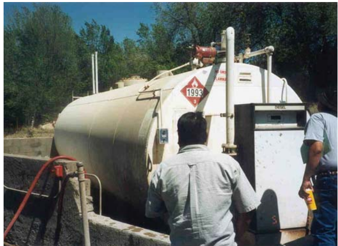
Upper left: Good example of secondary containment.
