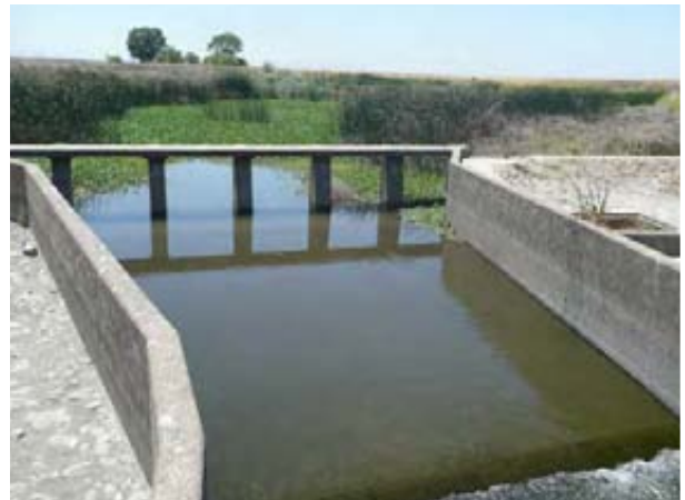
The Sand Slough Control Structure spills San Joaquin River water into the Eastside Bypass
