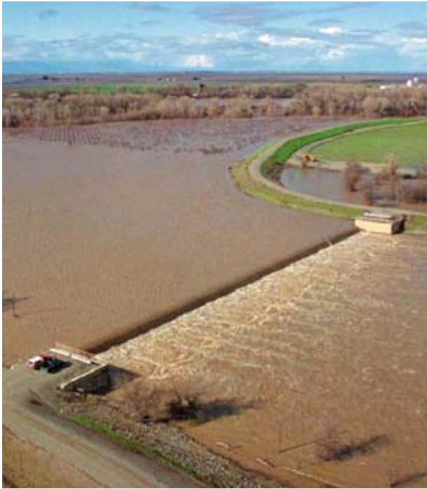
Moulton Weir spills water into the Butte Basin
