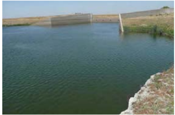
The drop structure on the Mariposa Bypass helps control the channel grade near its downstream end
