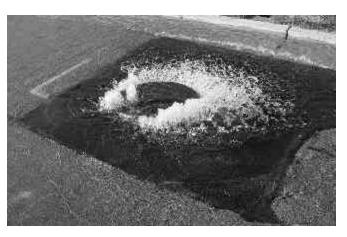
Some sanitary sewer overflows can occur at deteriorated manholes. (Photo courtesy of the Orange County Sanitation District.)
