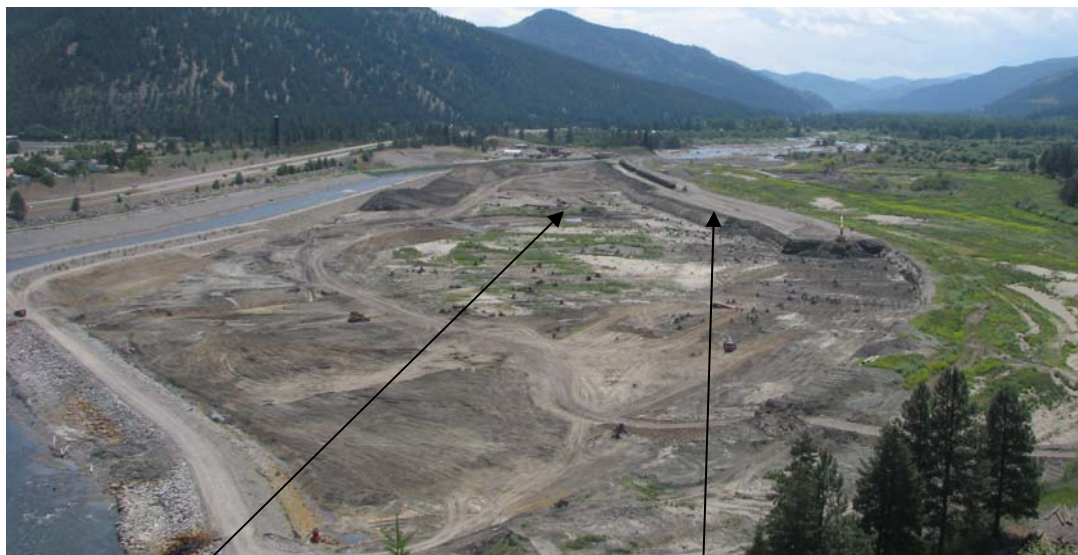
View of Project Area from Milltown Overlook, 7/7/09. The new Clark Fork River channel and floodplain are beginning to take shape. Notice the shortened rail line and excavation from underneath and around the former rail line footprint.
