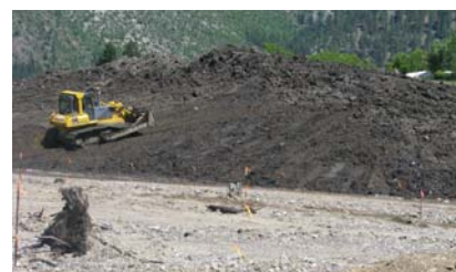
Stockpiling pre-dam native soils for later use in Site restoration.
