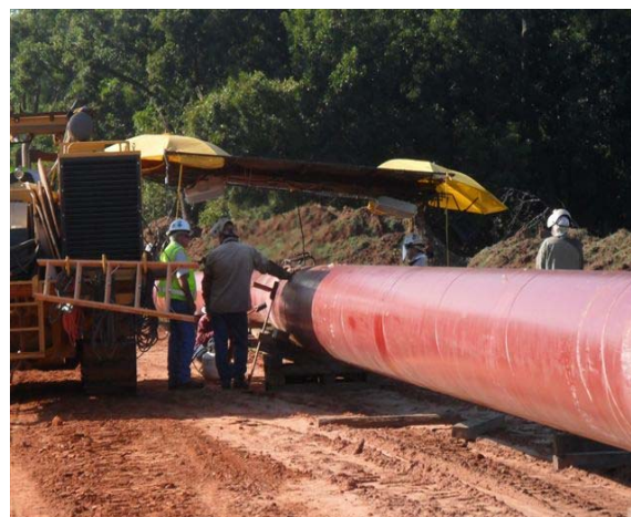
Figure ES-2 36-Inch-Diameter Crude Oil Pipe
